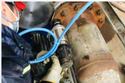
Extended Reaction Arm
